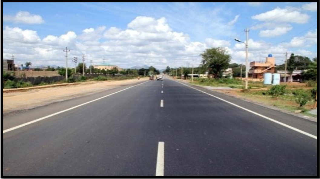
Photo 8: Strengthening by Cold Recycling Technology with RBI Grade-81: km 9.30 to 9.80, NH-206, Tumkur, Karnataka
