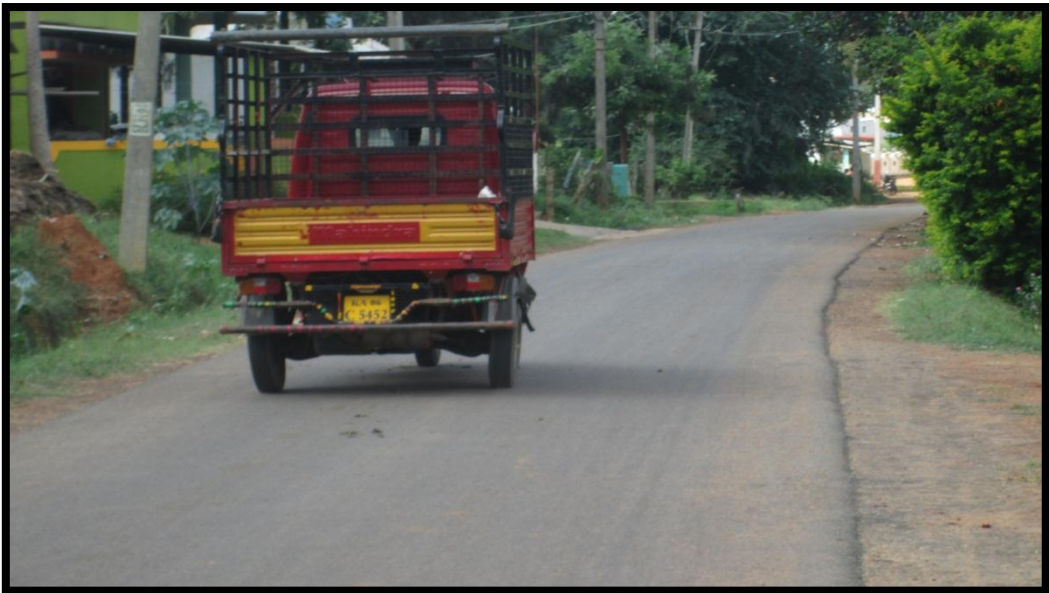
Photo 11: Rural Road: NH-206 to Basaveshwara Temple, Mattigatta Village Constructed with RBI Grade-81, Gubbi, Tumkur, Karnataka
