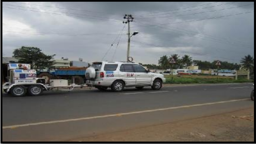
Photo 14: FWD Testing in Progress on Strengthening Stretch Constructed with RBI Grade-81
