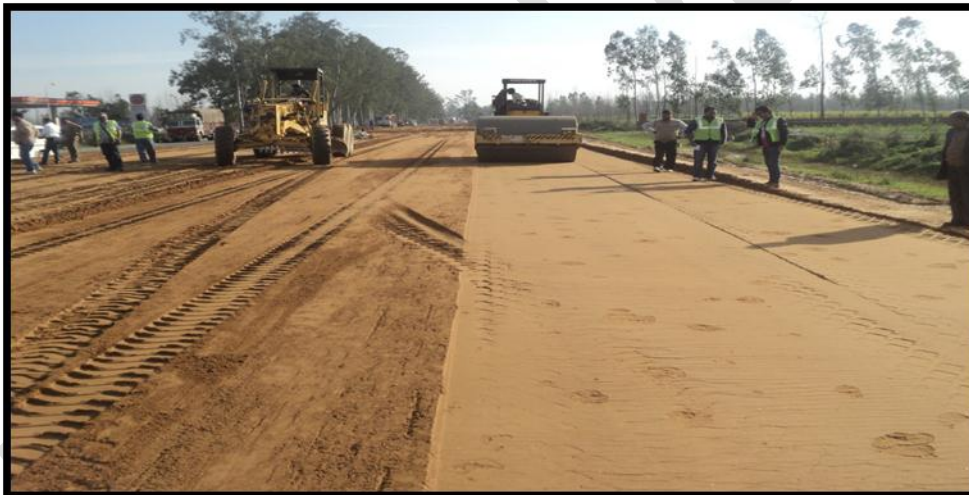
Photo 3.18: View of Initial Compaction of Construction Material
