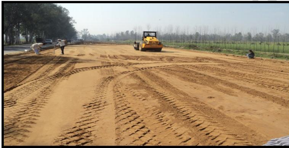
Photo 3.15: View of Preparing Subgrade
