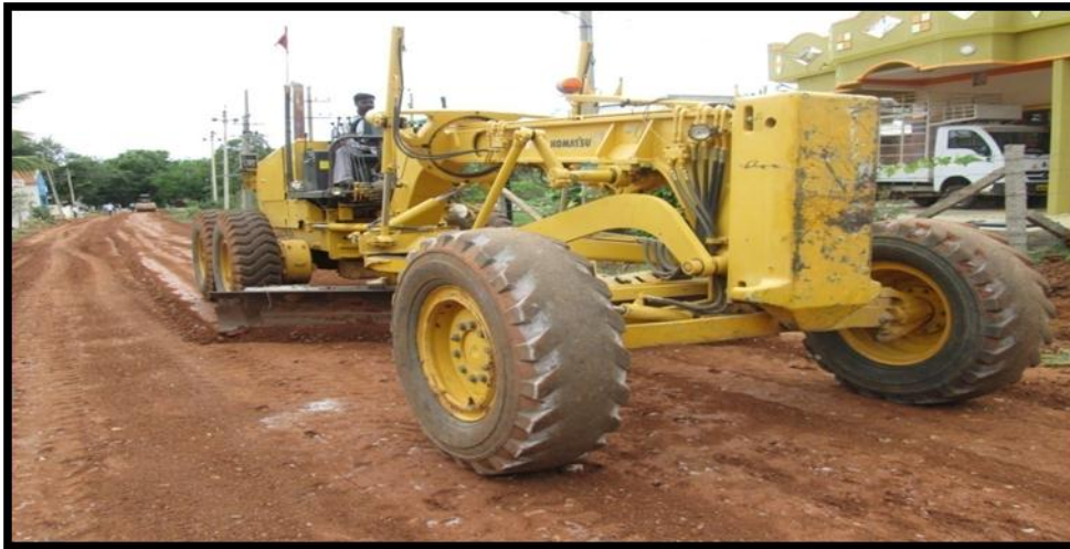
Photo 3.11: View of Grading in progress
