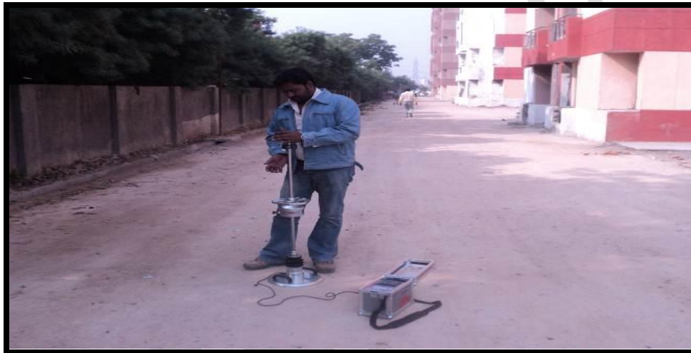
Photo 2.21: LWD Test in Progress
