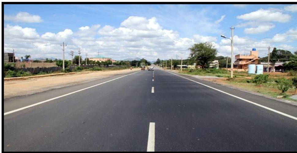
Photo 3.34: View of finished surface of Cold Recycling
