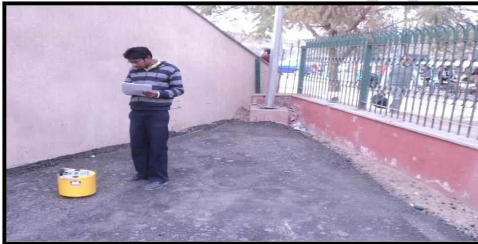
Photo 2.20: Geo Gauge Test in Progress
