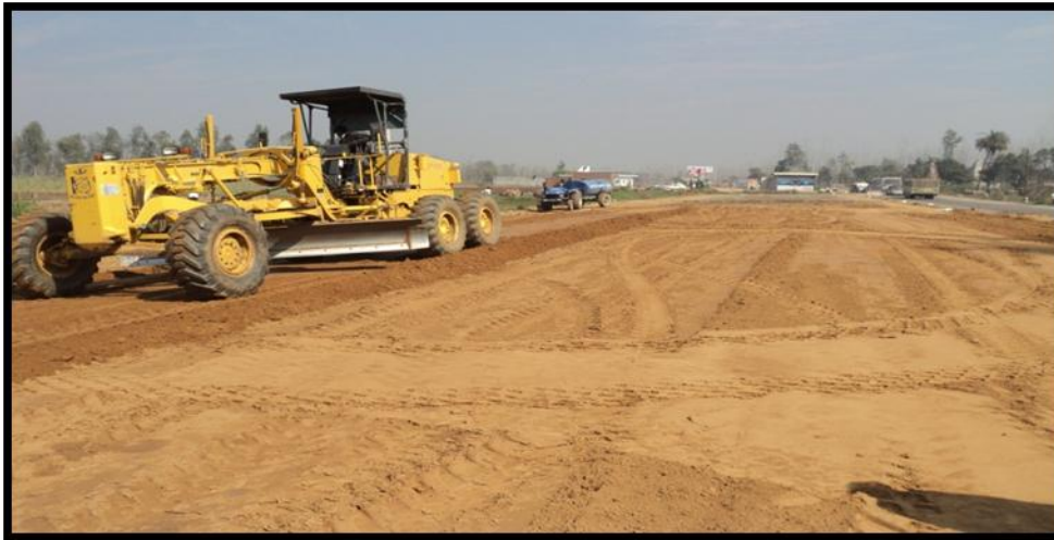
Photo 3.17: View of Spreading of Construction Material
