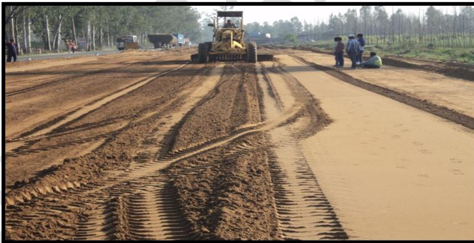
Photo 3.22: View of Grading of Stabilized Layer
