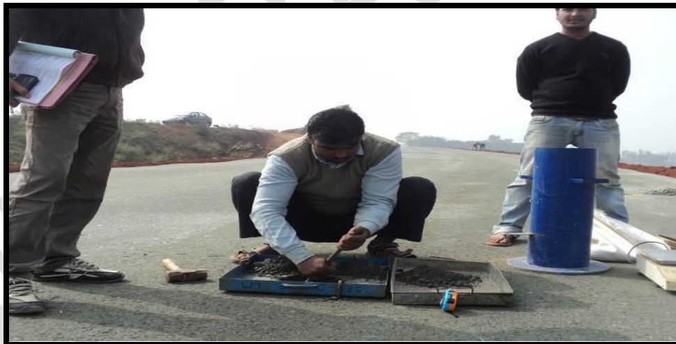
Photo 2.17: FDD Test by Sand Replacement Method in Progress
