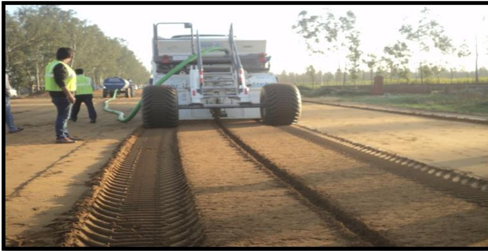
Photo 3.21: View of Stabilization by Stabilizing Machine of RBI Grade-81 layer
