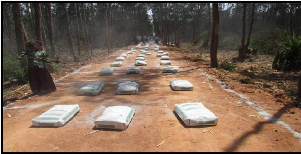
Photo 3.5: View of RBI Grade-81 bags laying
