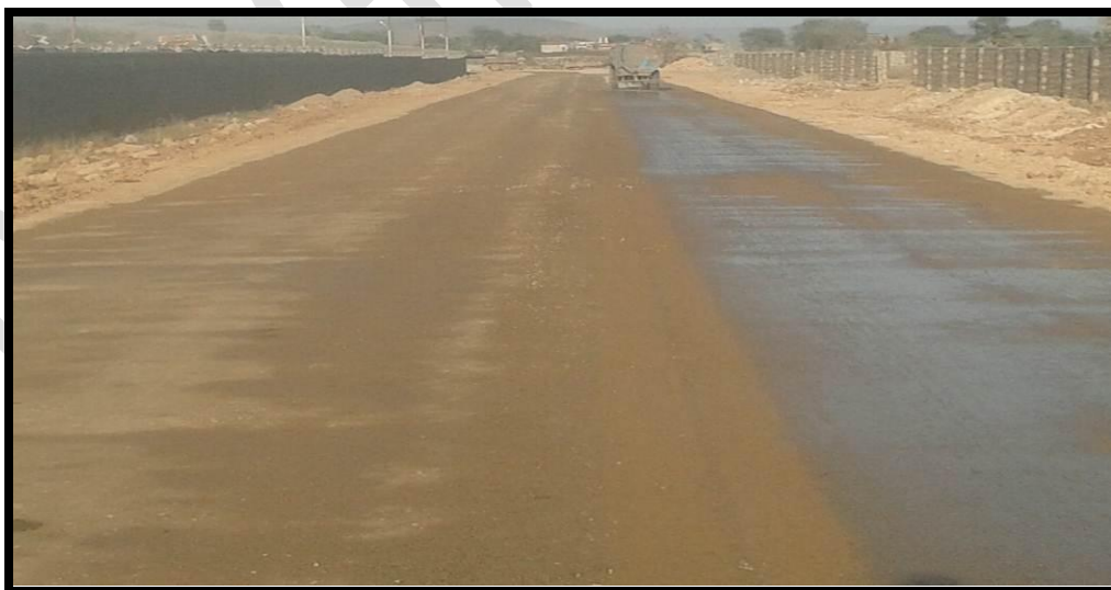
Photo 3.33: View of Curing in progress
