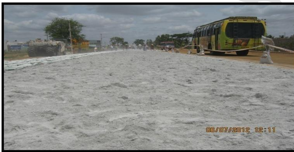
Photo 3.28: View of Spreading of RBI Grade-81
