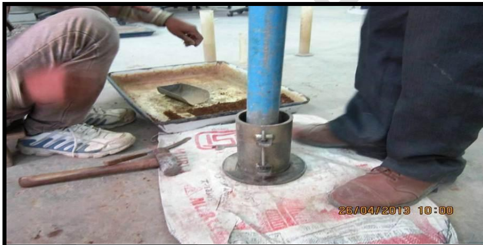
Photo 2.6: Modified Proctor test in Progress
