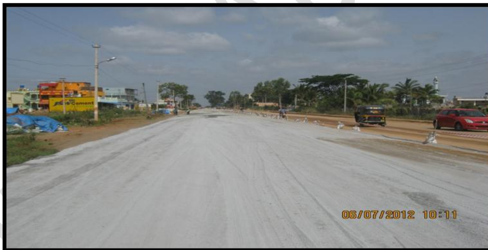
Photo 3.26: View of Spread Stone Dust on Existing Pavement
