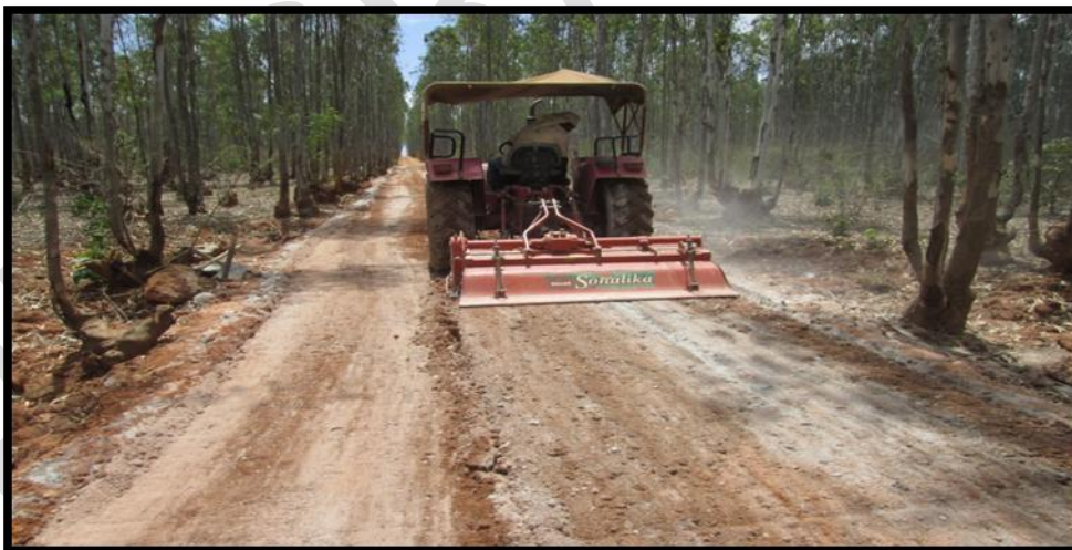
Photo 3.10: View of Wet Mixing by Rotavator
