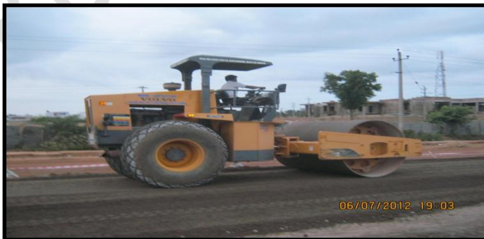
Photo 3.31: View of Compaction in Progress
