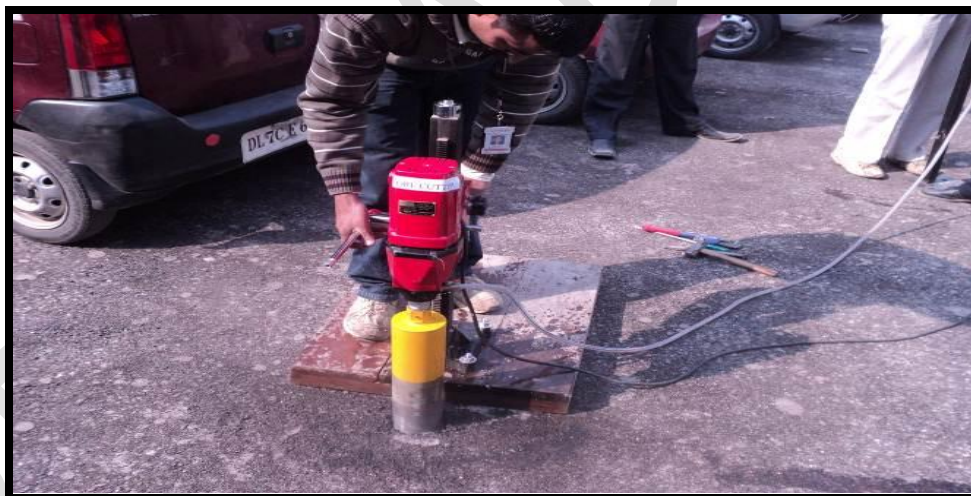
Photo 2.18: Core Cutting in Progress
