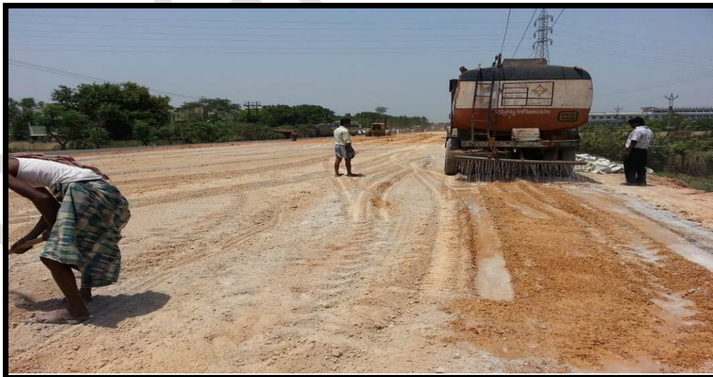
Photo 3.8: View of water addition
