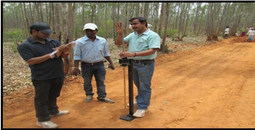
Photo 3.3: View of Checking of Existing Subgrade compaction by DCP
