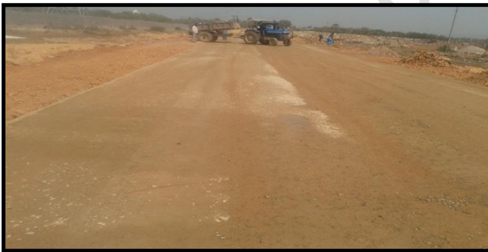
Photo 3.38: View of Final Surface
