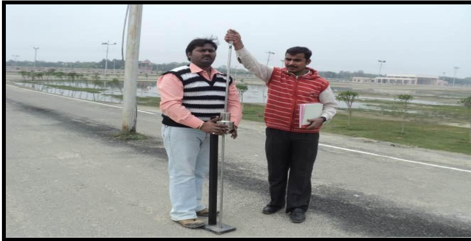
Photo 2.19: DCP Test in Progress
