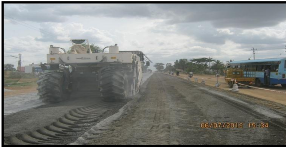
Photo 3.29: View of Milling & Mixing with Stabilizing Machine
