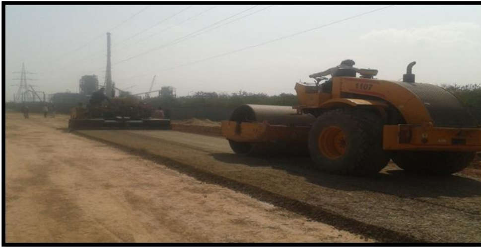
Photo 3.37: View of Compaction
