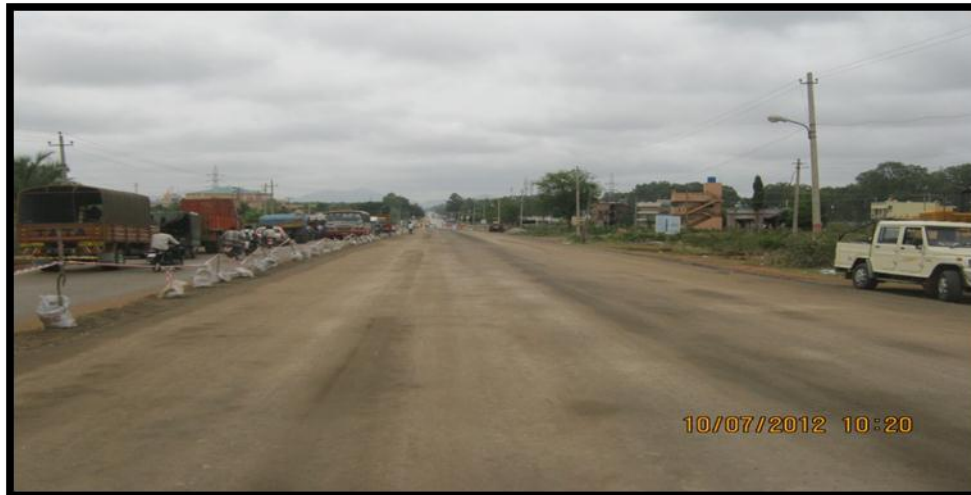
Photo 3.32: view of Completed Cold Recycling
