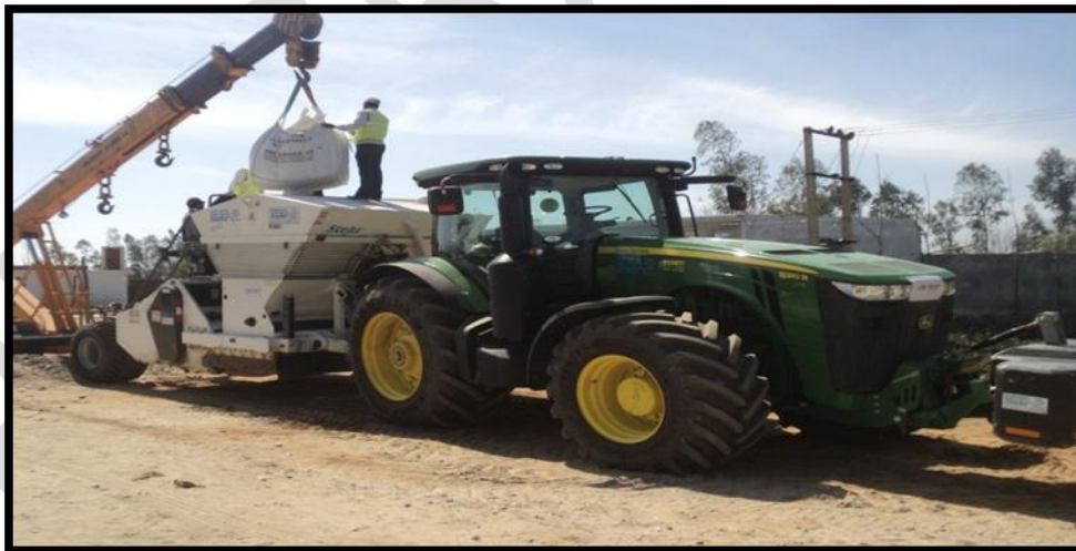
Photo 3.20: View of Filling of RBI Grade-81 in Stabilizing Machine
