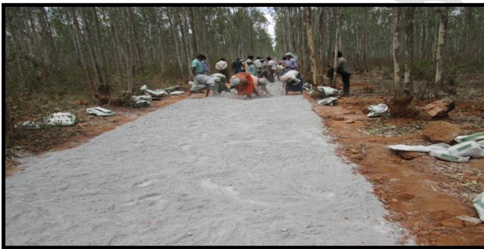
Photo 3.6: View of RBI Grade-81 Spreading
