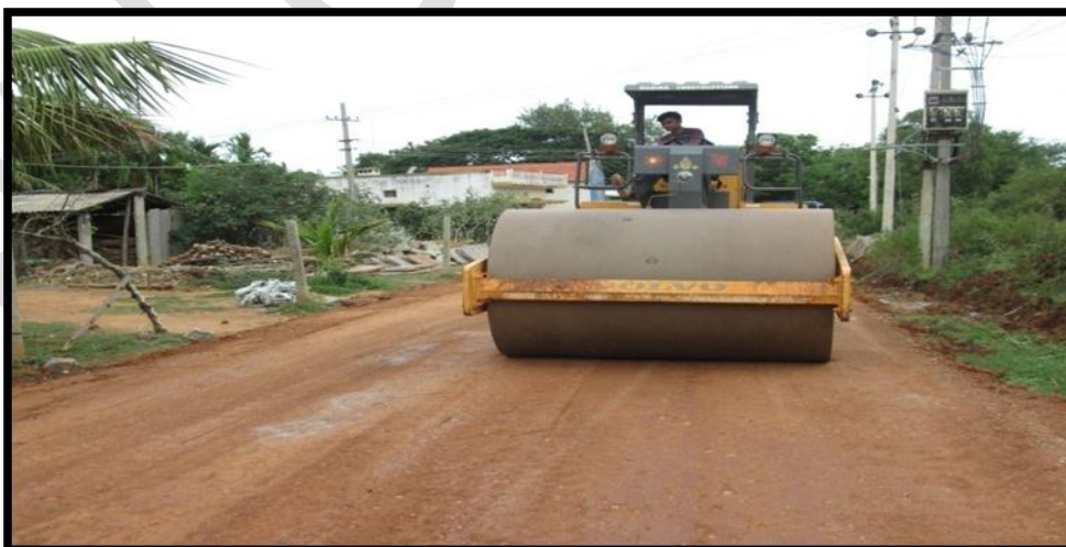
Photo 3.12: View of Compaction in progress
