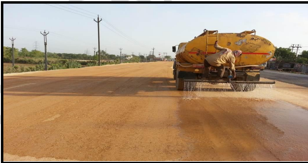
Photo 3.14: View of Curing of Stabilized Layer
