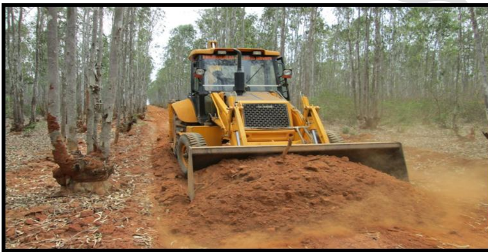
Photo 3.4: View of Spreading of Construction Material for Stabilized Layer
