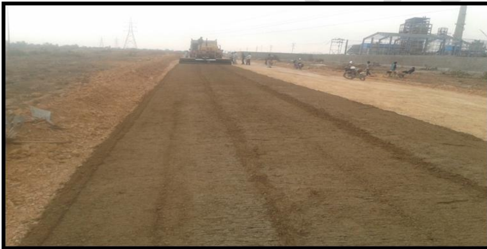
Photo 3.36: View of Laying of RBI Grade-81 layer by Paver
