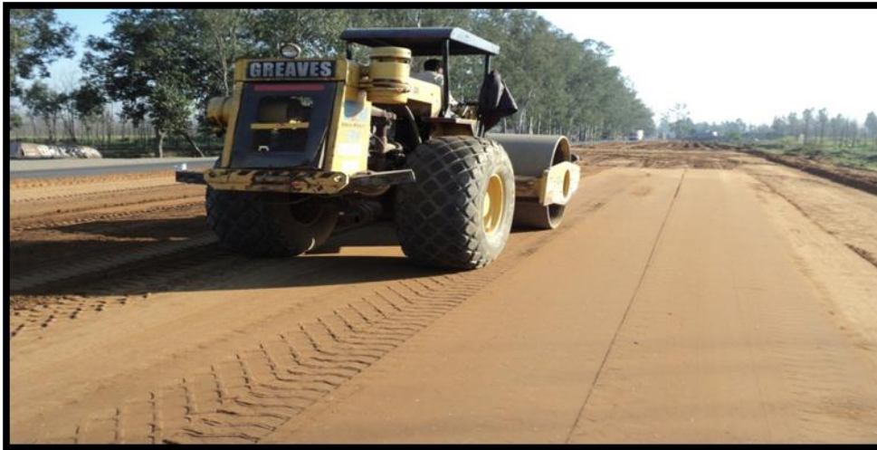
Photo 3.23: View of Compaction of Stabilized Layer
