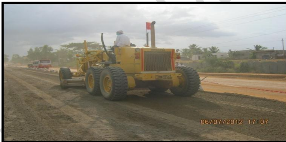
Photo 3.30: View of Grading of Recycled layer in progress
