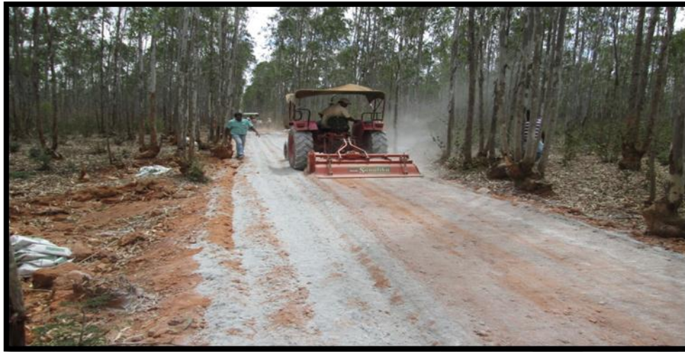
Photo 3.7: View of Dry Mixing with Rotavator
