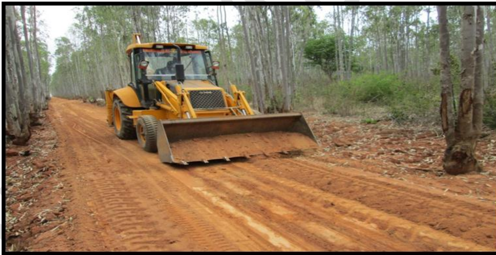
Photo 3.2: View of Bed Preparation in Progress
