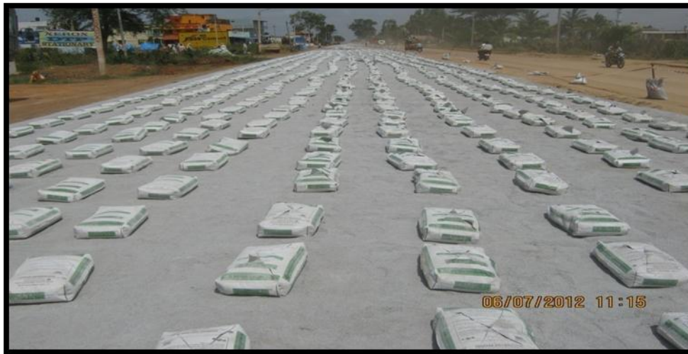
Photo 3.27: View of Laying of RBI Grade-81 bags
