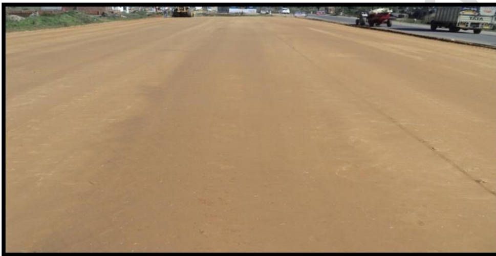
Photo 3.24: View of Final Compacted Stabilized Layer
