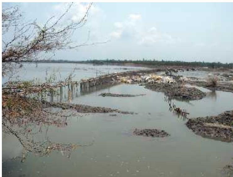
Breaching of the Embankment in Sonakhali Sundarbans during Cyclone Aila 119
