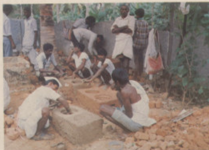
Fig 35: Construction of Wood efficient burning chullahs.
