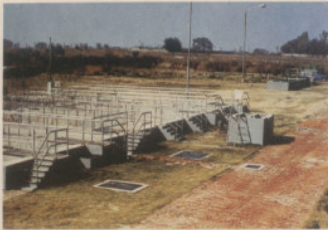
Fig 26: Sewage Treatment Plant at Belur.
