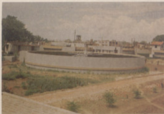
Fig. 24: Sewage Treatment Plant at Banaras Hindu University established under Ganga Action Plan.
