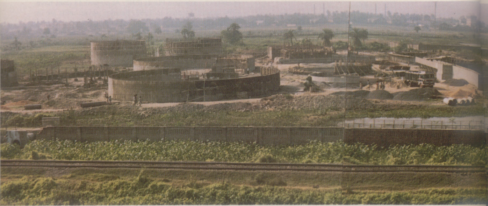
Fig. 45 Panoramic view of a sewage treatment plant at Gardenreach, Calcutta
