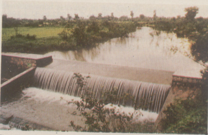
Fig. 40 Moisture conservation through check dams
