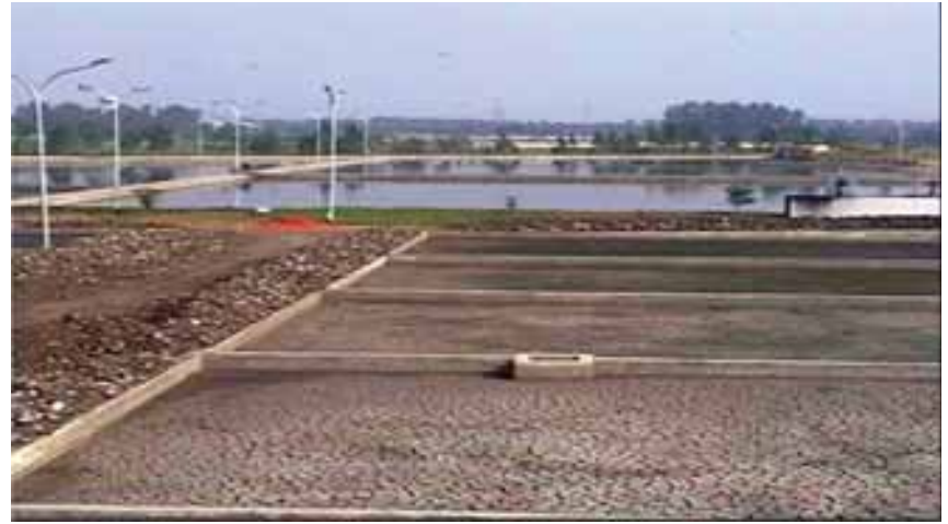
Fig-61. Sewage treatment plant at Saharanpur, Uttar Pradesh
