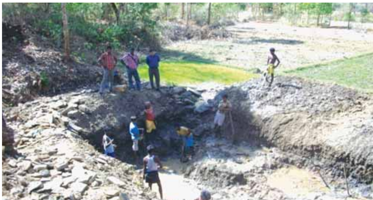
Fig-30. Excavation of pond at Khunti site in Jharkhand
