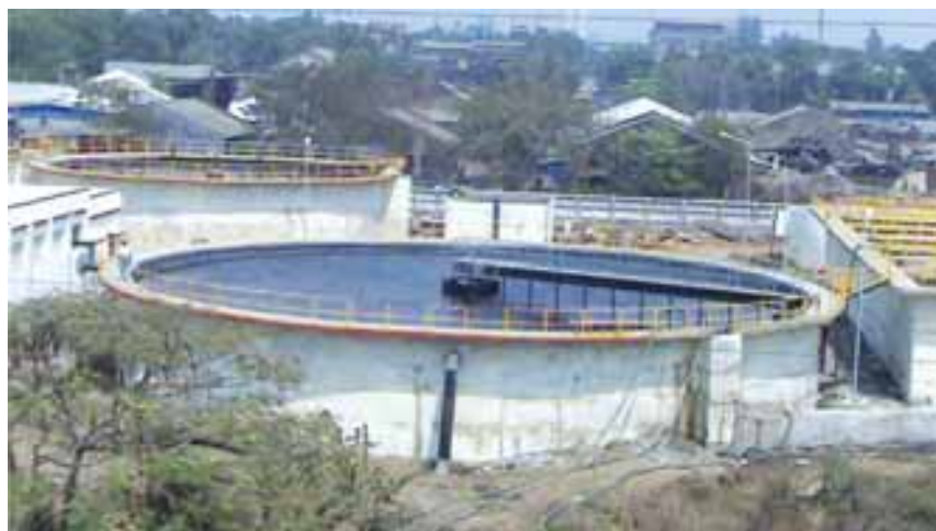
Fig. 47 : Common Effluent Treatment Plant Clarifier at Taloja, Navi Mumbai
