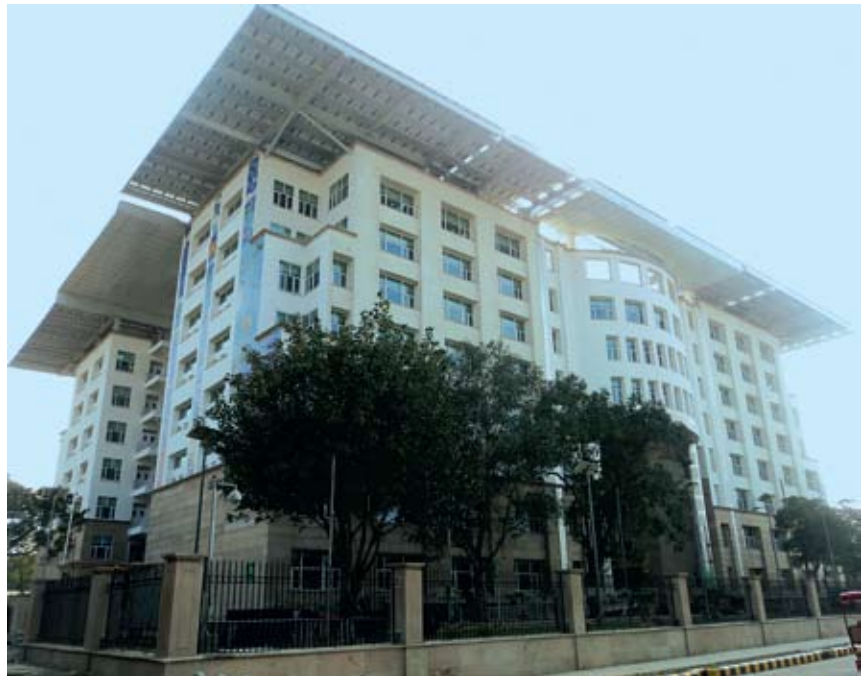
Fig-60. Ministry's new office building at Jorbagh Road, New Delhi
