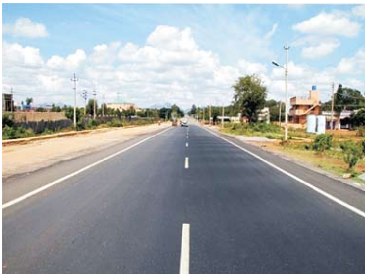
Fig-28. Road constructed using Cold Recycling Technology: 9.30 to NH-206, Tumkur, Karnataka
