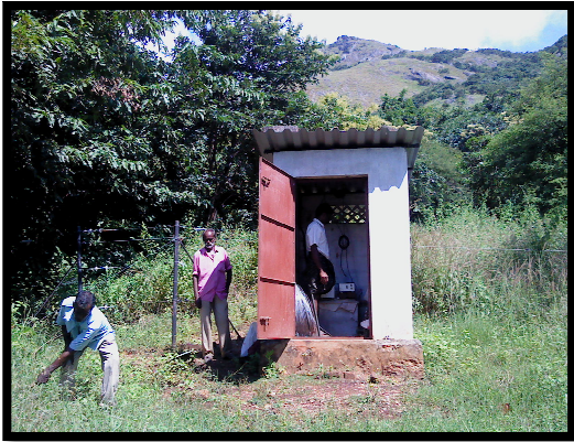
Fig. 4.3: Power fence along the track
