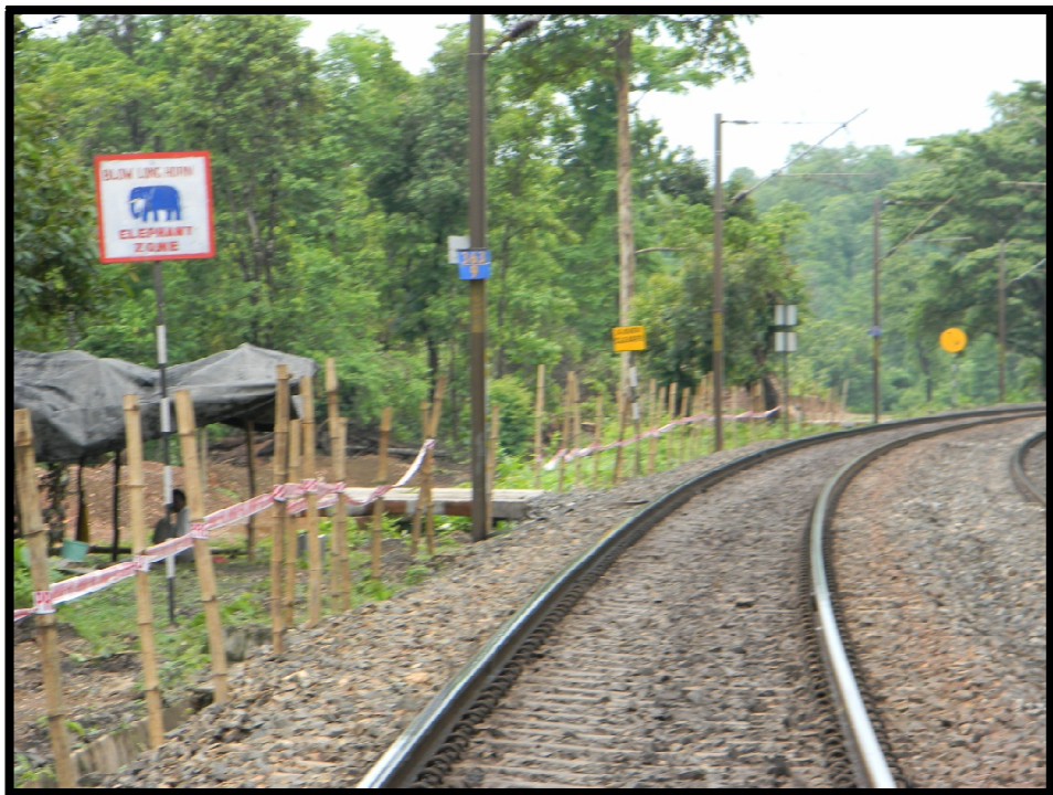
Fig. 3.12 Caution signage along the railway track in accident prone area between Posotia and Manoharpur section in Kolhan FD
