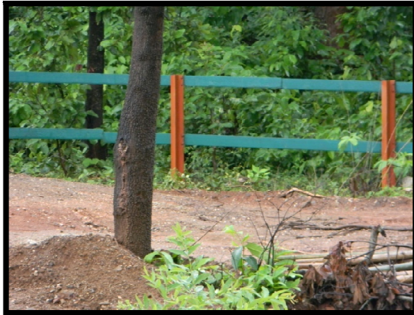
Fig 5.1: Old rail fencing to prevent elephant movement in Jharkhand
