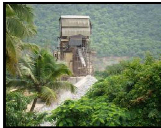
Fig. 3.18: Malabar cement factory
