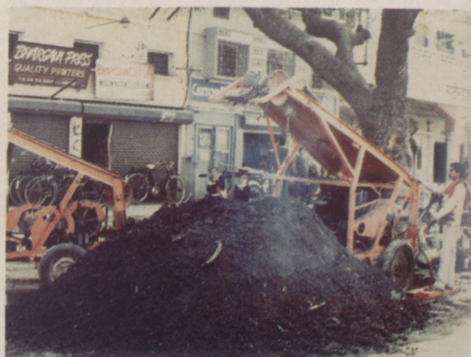
Fig 18: Ganga Action Plan—Cleaning of Sewer lines.
