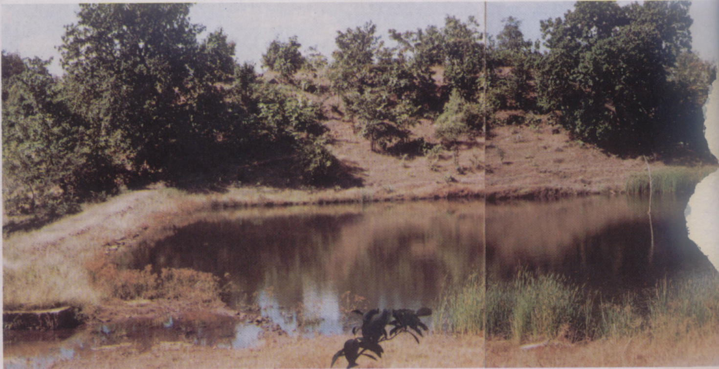
Fig. 45 Earthen bunds built under Technology Mission and Yojna Mandal-a multi-purpose project
