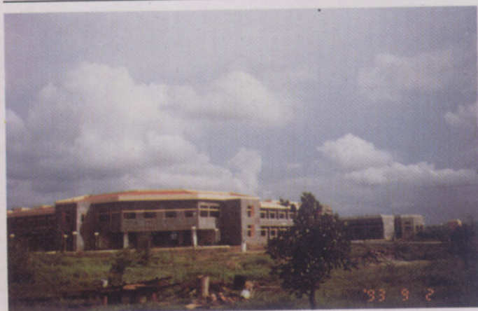
Fig. 84 The laboratory building of TFRI, Jabalpur
