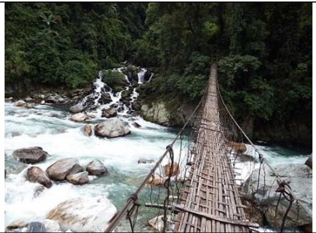
Dav river near suspension bridge, Dav Basti
