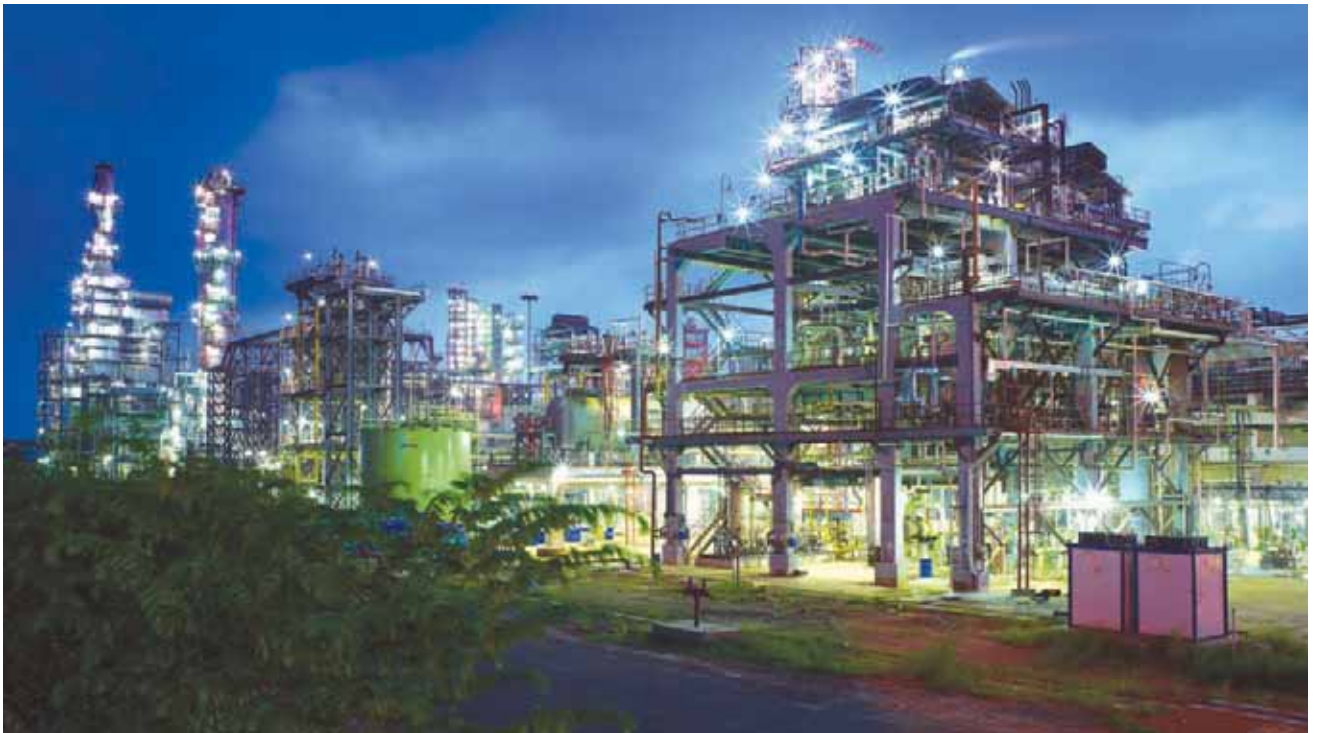
Bharat Petroleum Refinery, Kochi
