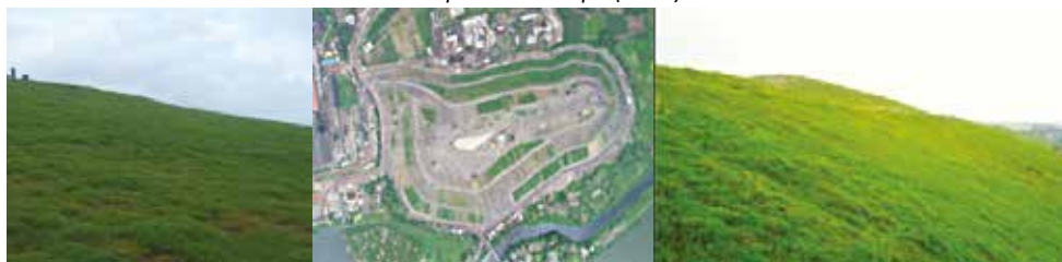
Dump Site at Dhapa (Now)
