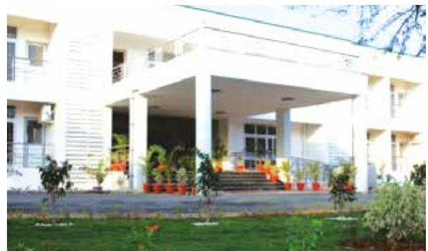
Construction of Executive Hostel under JICA project in CASFoS, Coimbatore.
