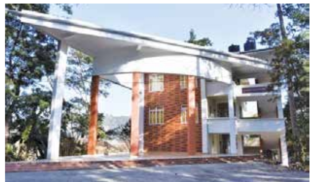
Newly Constructed Academic Building, SFTI, Aizwal, Mizoram
