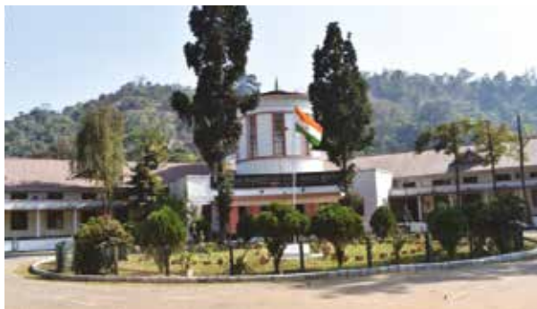
Academy Building, CASFoS, Burnihat, Assam
