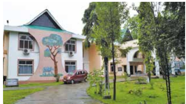
Newly constructed Academic cum Administrative Building, SFTI, Makum, Assam
