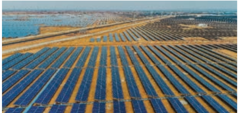
Figure 6.3: Kurnool Solar Park, Andhra Pradesh, with a capacity of 1,000 MW is operational since March, 2017
