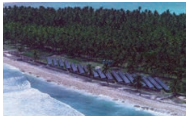
Figure 6.7: 100 KWp grid interactive solar power plant, set up on Kalpeni island, Lakshadweep.
