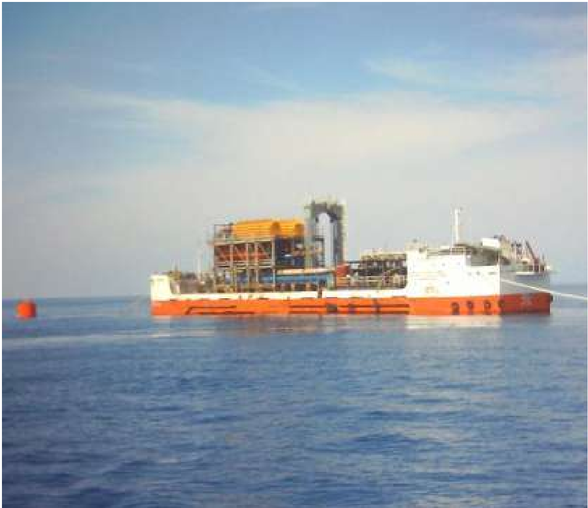
Figure 10: View of the Barge Mounted Desalination Plant
