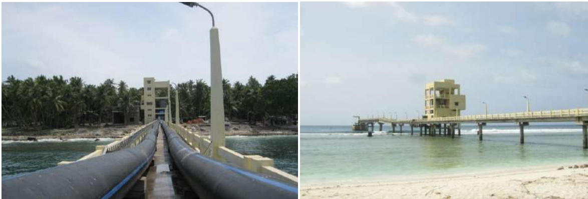
Figure 5: Desalination Plant at Minicoy & Agatti Islands
