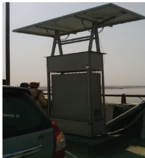
RTWQM Station at Kachlaghat ( U.P.)
