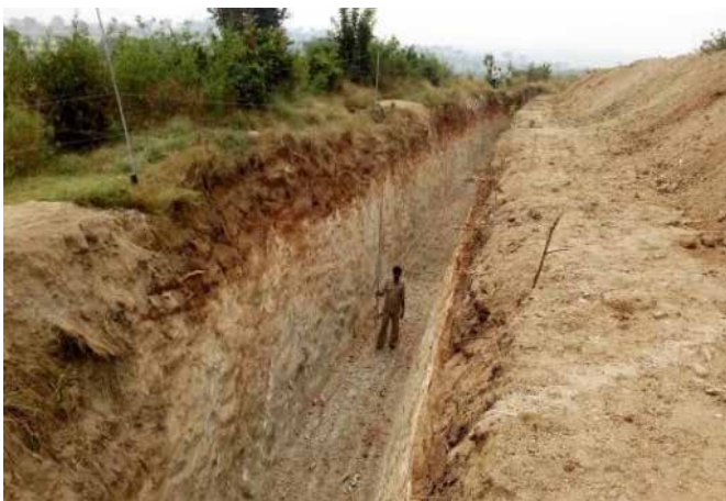
Photos 3: Upgraded Elephant Proof Trench (EPT) with dimension of 3x3x1.5 meters at
