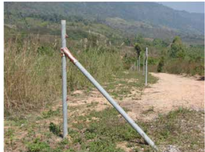
Fig 3 A properly installed and well maintained Solar Power Fence
