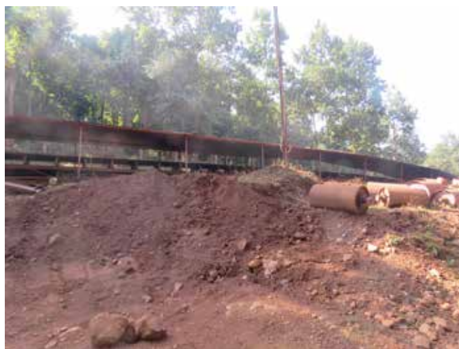
Fig. 12: 12.38km long conveyor belt of Daitari iron ore mine in Similipal-Satkosia corridor
