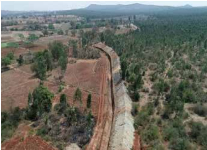
Photos 1: Elephant Proof Trench (EPT) of 3x2x1 meter dimension at Bolegowdana Katte Beat of Omkara Range.
