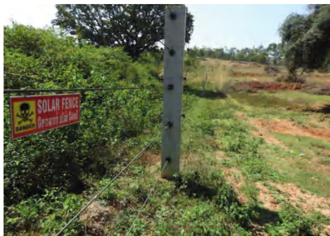
Solar fence to mitigate elephant conflict at Hosur Forest Division, Tamil Nadu
