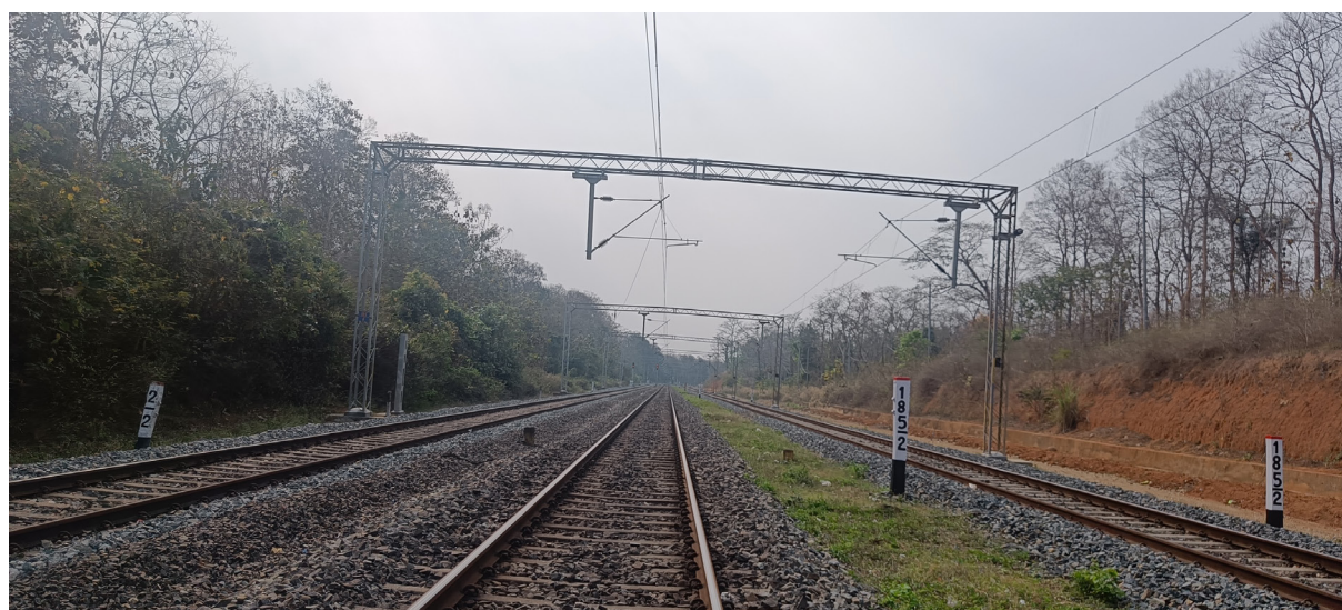
Figure 30: The space between parallel tracks should also be covered with the level crossing material recommended at elephant crossing sites.
