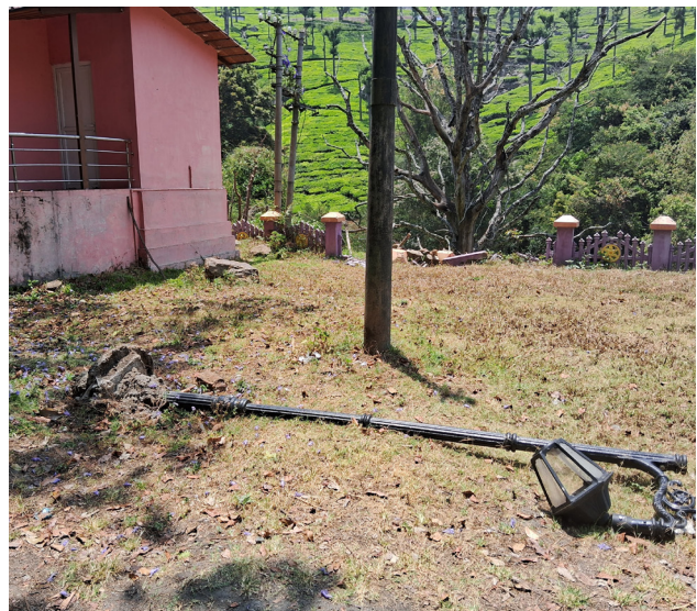
Figure 11: Damage by elephants at Runnymede station on the Kallar – Ooty railway line.
