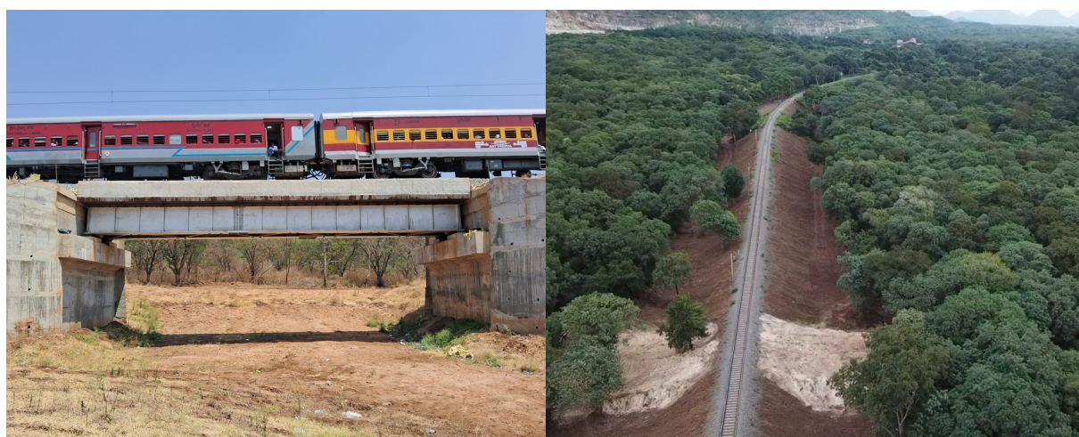
Figure 5: Mitigation structures in Madukkarai Forest range. Left – Underpass of 10 x 18 m dimension; the structure requires installation of light and sound barriers on both sides. Right – level crossing ramp, the structure requires upgradation to make a rubberized level crossing on the track.
