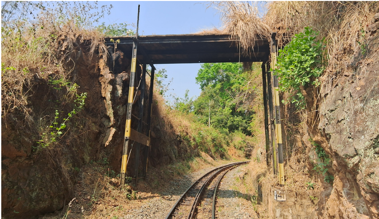
Figure 12: An Indian gaur fell from the overbridge and died at bridge no. 41 ( 11^{\circ}20'39.23''\text{N} , 76^{\circ}51'14.19''\text{E} ).
